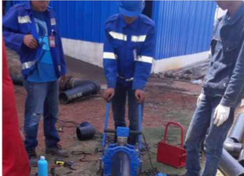
PIPING ON SITE
