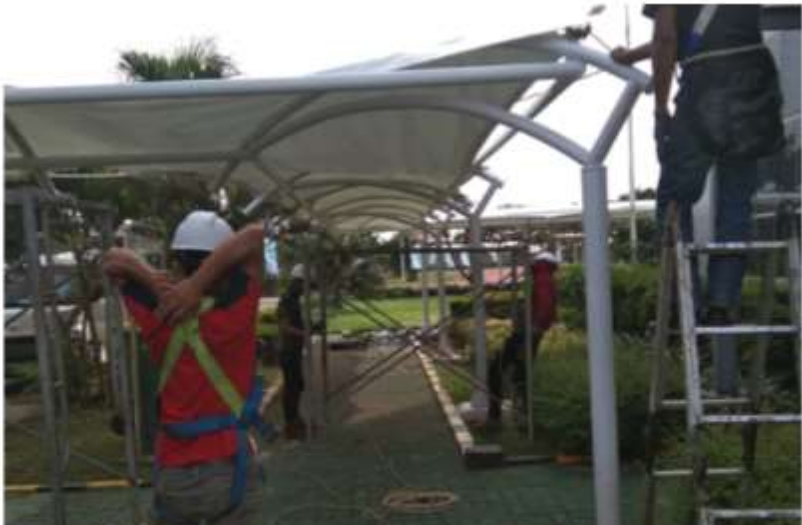
JOB Canopy Membrane at Power Plan Indramayu
