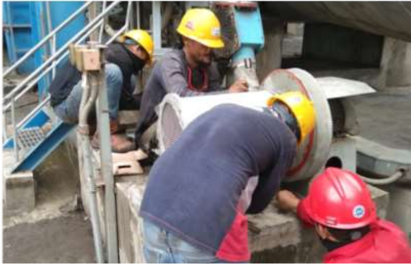
ASSY on Site FILTER AIR ID FAN
