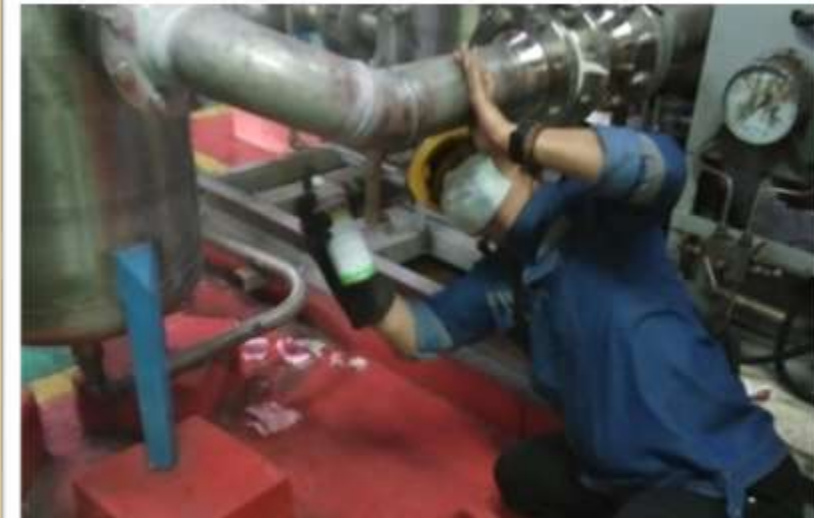
NDT Process Job Site at Indramayu Power Plan
