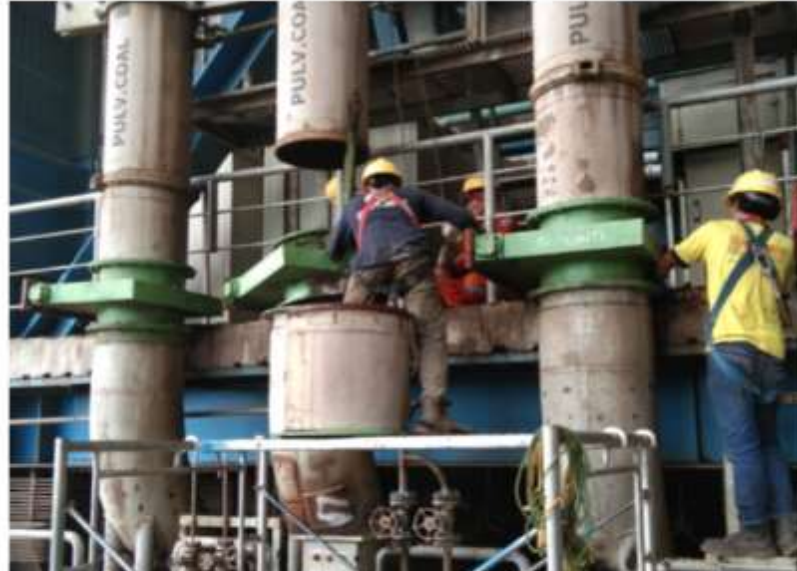
Assy ORRIFICE MILL VALVE BURNER
